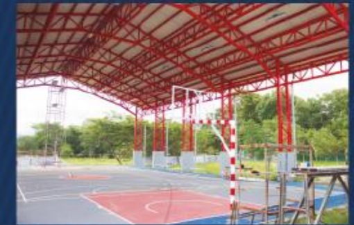
Obras Recreativas Campus Coto
